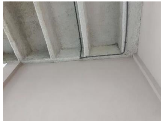
V0000 (None), Structure, Fireproofing, Pool Exterior Walls (Location #: 16)
