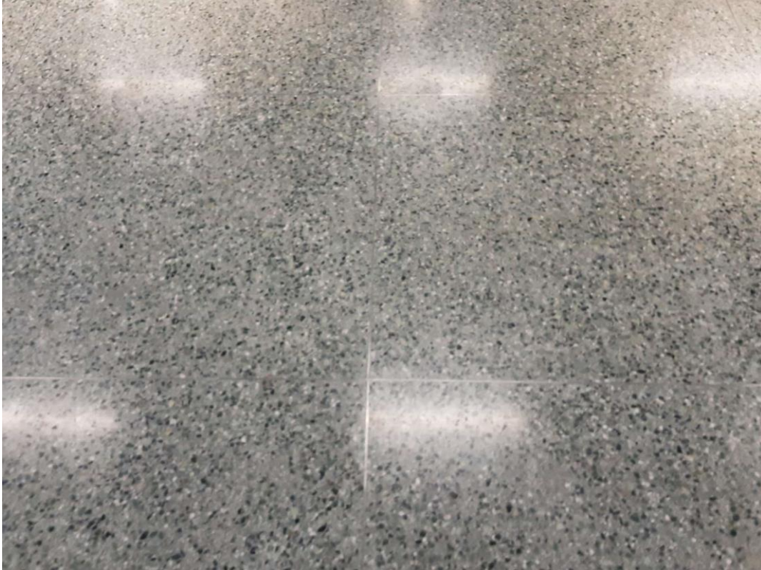
V9500 (Presumed Asbestos), Floor, Terrazzo, Foyer (Location #: 15)
