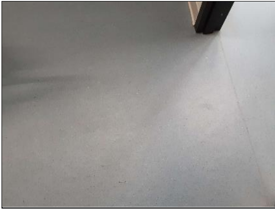
V0000 (None), Floor, Vinyl Sheet Flooring, Stairway To Stage (Location #: 5)
