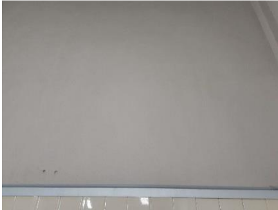
S0011A (None), Wall, Texture Coat, Pool Exterior Walls (Location #: 16)
