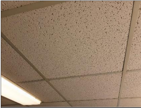
V0000 (None), Ceiling, Ceiling Tiles (lay-in), Men's Washroom (Location #: 10)
