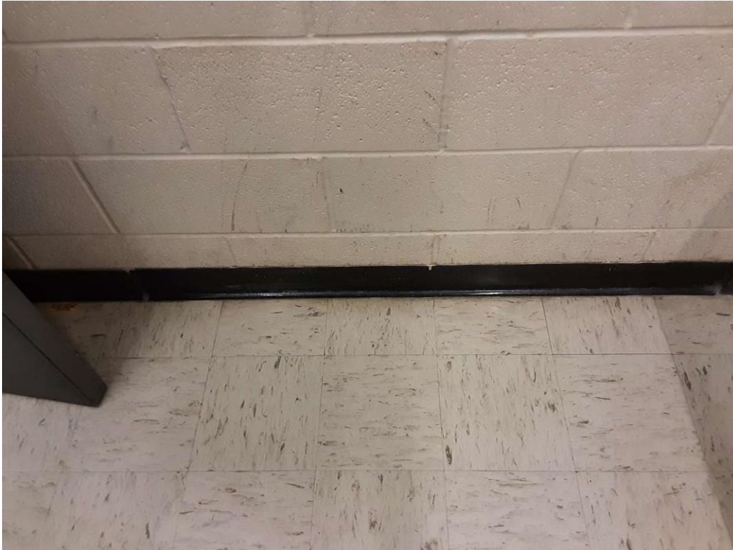
S0004A (None), Wall, Base, Adhesive/mastic, Storage Room (Location #: 3)
