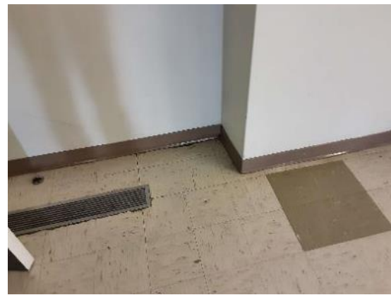
S0001B (None), Wall, Base, Adhesive/mastic, Auditorium (Location #: 1)
