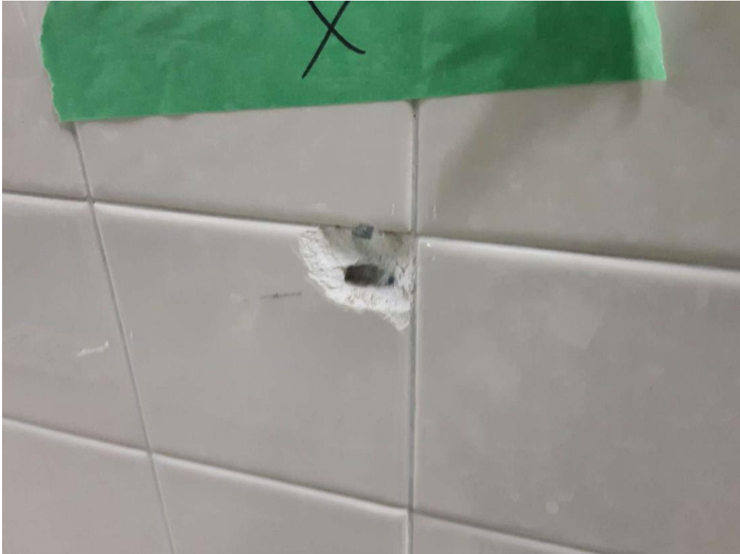
S0010A (None), Wall, Ceramic Tile Thin-Set, Pool Exterior Walls (Location #: 16)
