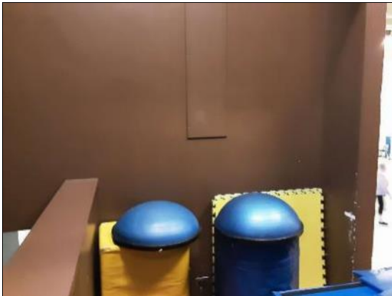
S0002A (None), Wall, Plaster, Stage (Location #: 2)
