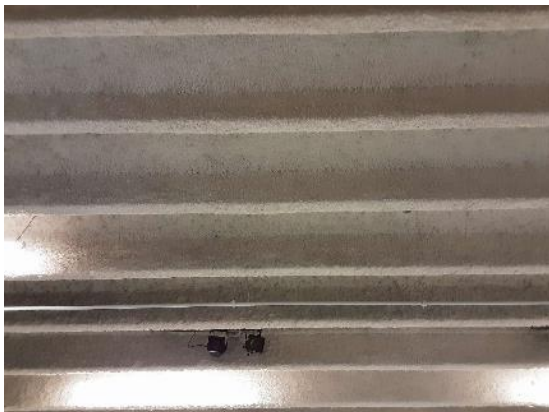
V0000 (None), Structure, Beam, Deck, Acoustic spray, Auditorium (Location #: 1)
