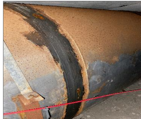
V0000, (None), Duct, blackish grey mastic, Crawlspace (Location # 20)
