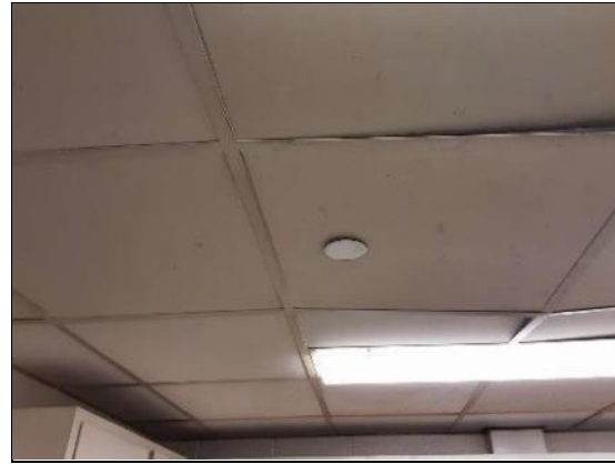
V0000 (None), Ceiling, Ceiling Tiles (lay-in), Kitchen (Location #: 9)
